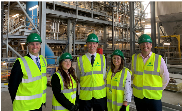
Members of the three charities took a tour to explore inside the Beddington Energy Recovery Facility.
